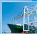
LAEM CHABANG PORT Thailand's main port with world class facilities and services strategically locates in the fastest growing industrial area.
