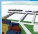
RANONG PORT Gateway to the Southern-west coast to accommodate trade expansion in South Asia.
